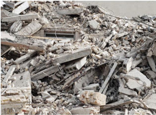
Gambar 3. Sisa Material Bongkaran Beton
